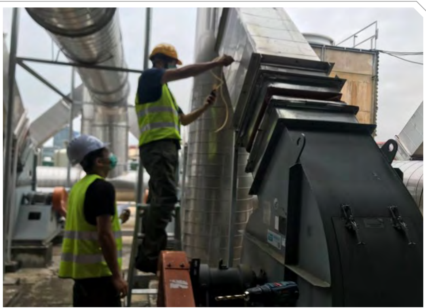
Inspection of ventilation devices
