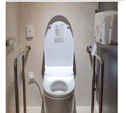
Accessible facilities in Wistron's work environment
