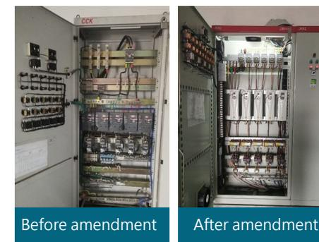
Chengdu Plant: Changed cooling tower fan into inverter system
