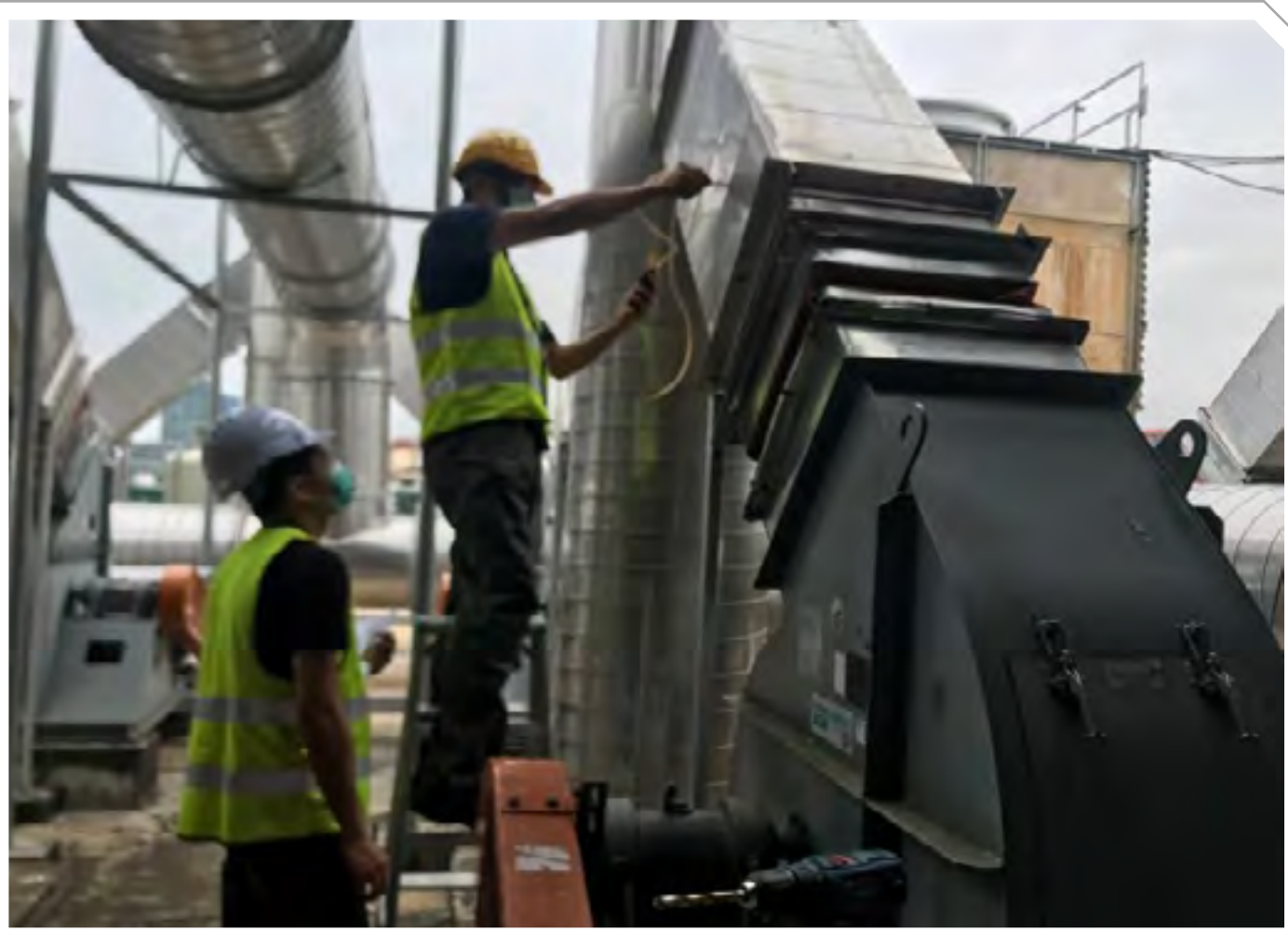
Inspection of ventilation devices
