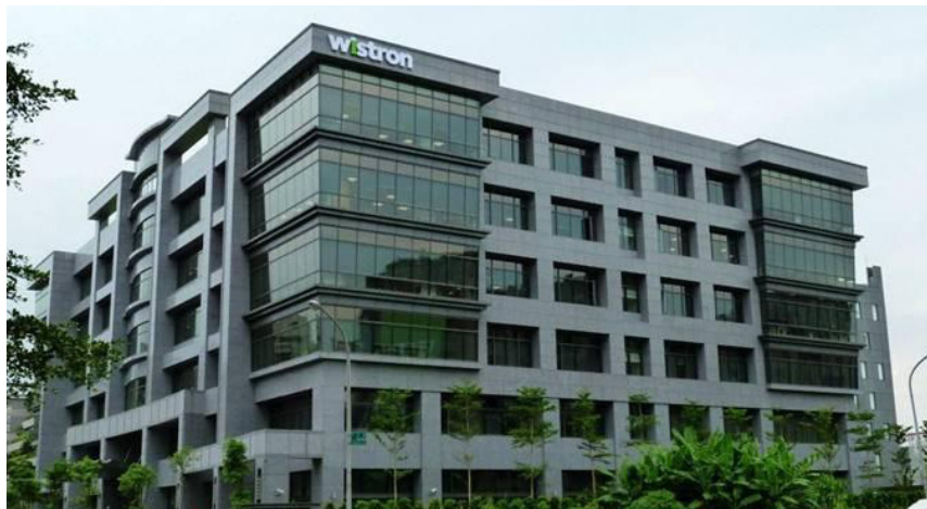
Greening was adopted as the rooftop insulation solution for the Neihu Headquarters building
