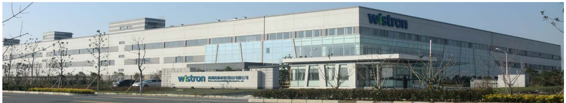
Wistron Advanced Material Kunshan PCR Refining Plant
