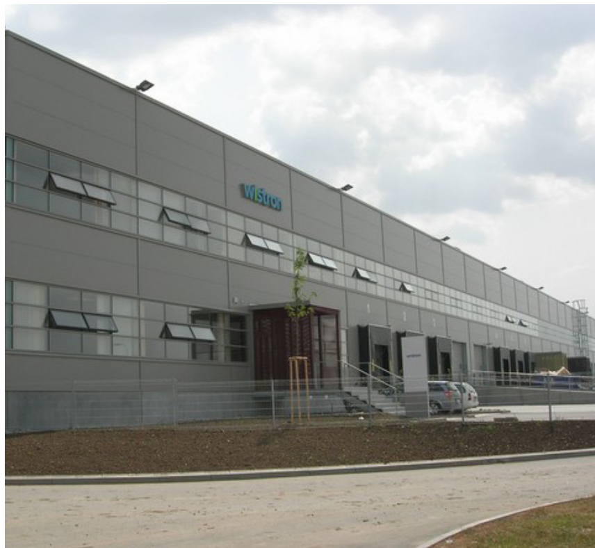
Czech Plant - Introduction of More Efficient Ecological Heating Systems One of initiative for year 2012 in energy saving field is optimization of building heating together with hot water warming. New campus is using ecologic way of heating and water warming. Hot steam from heating plant is distributed to surrounding plants. Hot steam is converted to hot water. WCZ plant is connected to this heating system and will use this ecologic heating way for heating during winter 2012/2013
