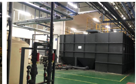
● Taizhou Plant - Exterior of the wastewater treatment station
