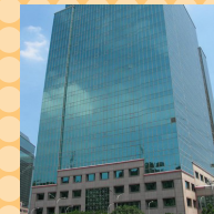
Hsichih Office Complex
