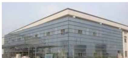
Chengdu Plant - Uses Low-emissivity energy-saving glasses.
