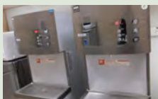
Used timer controlled energy-saving water dispenser.
