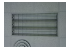
Chengdu Plant - Substituted traditional T8 lighting tubes with the T5 type.
