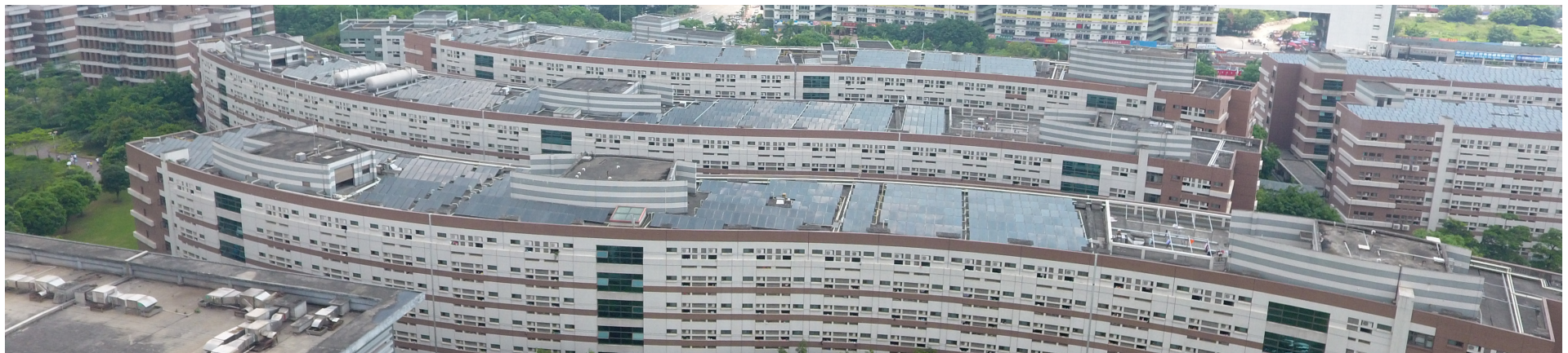
● WZS_ Solar water heaters for employee dormitories
